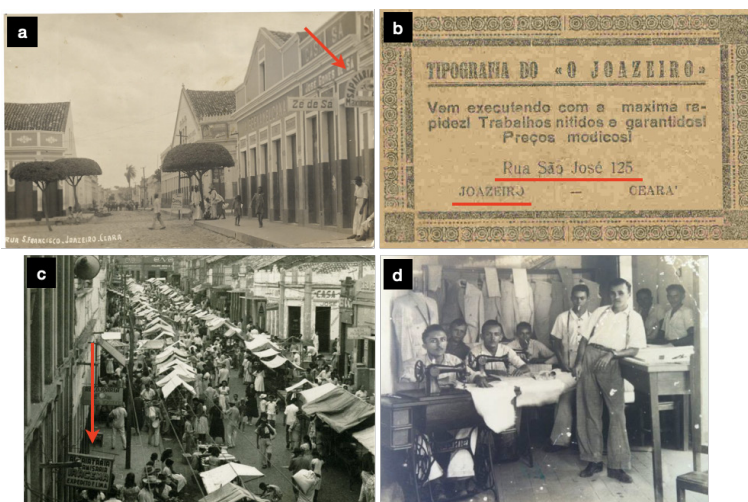
Figure 2 – Examples of workshops installed in the city center
