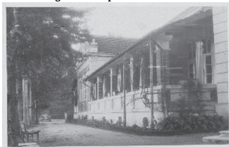
Figura 7 - Hospital Santa Catarina
