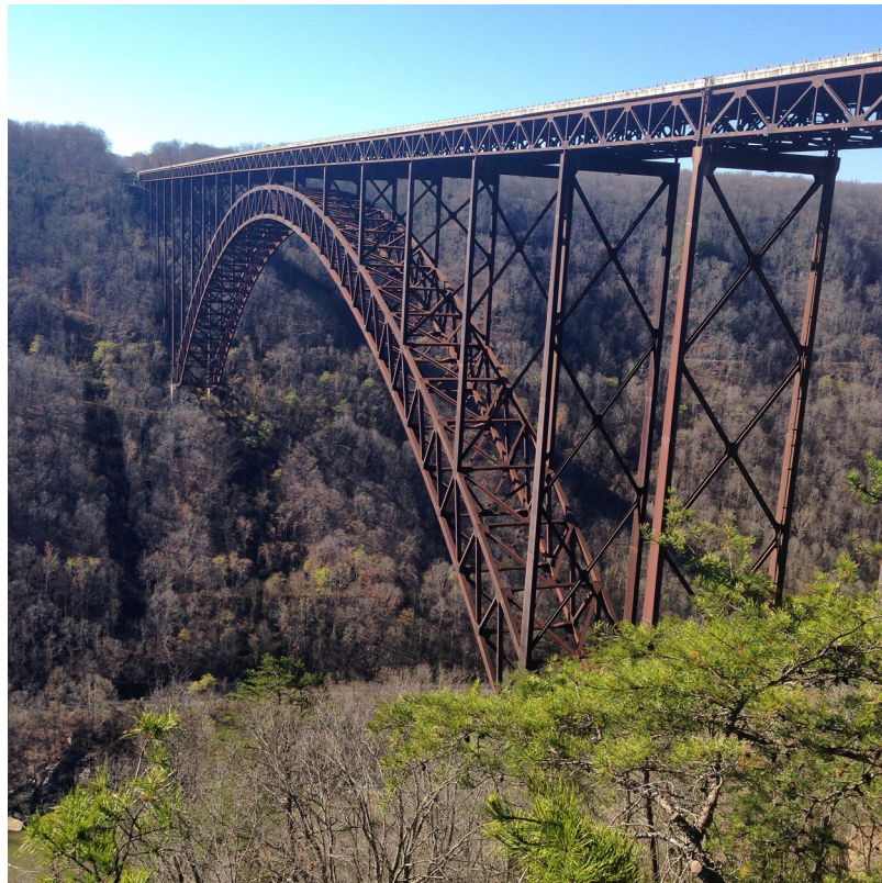
Figure 3: New River Gorge Bridge, West Virginia.
